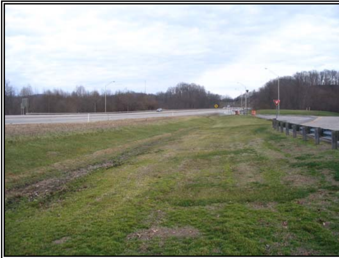
I-79 Rest Stop Monitoring Site Looking North
