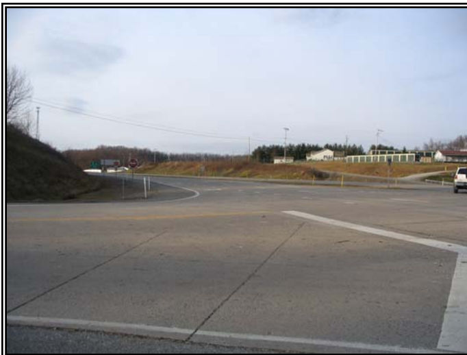
Childer's Run Monitoring Site Looking West
